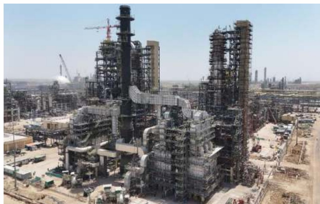
Pic1: Crude Distillation Unit construction at HRRL
